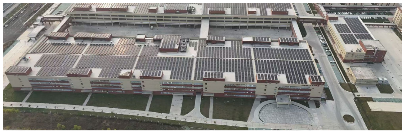
Bird's-eye view of PV power generation in Hefei Park
