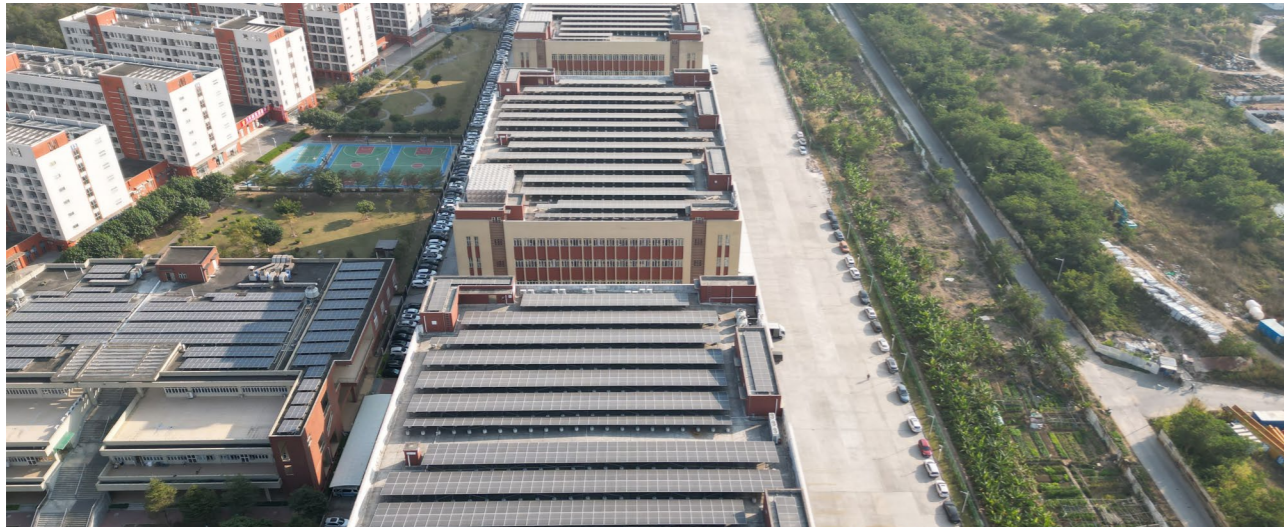
Bird's-eye view of PV power generation in Nanping Park
