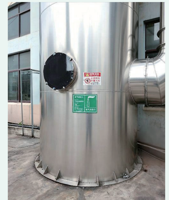
Decontamination Furnace Waste Gas Discharge Outlet Signage (After Rectification)
