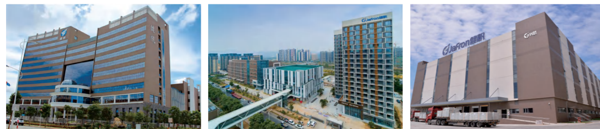
Jafron Science and Technology Park South Campus
