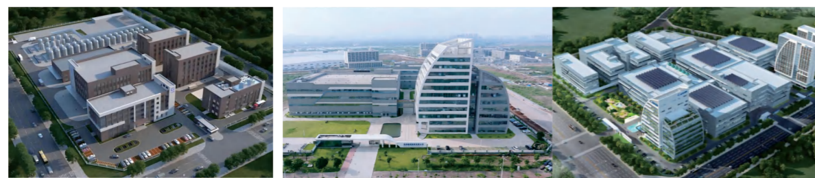
Jianshu New Materials Production Base (under development)
