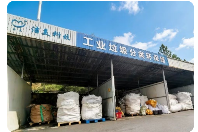
Waste Sorting Area
