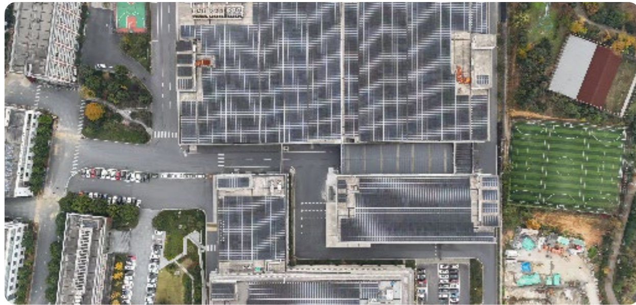
Rooftop distributed photovoltaic power generation project
