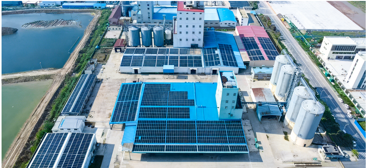
The PV project at Sheyang Liuhe Feed Co., Ltd. was successfully connected to the grid on June 15, 2025.
