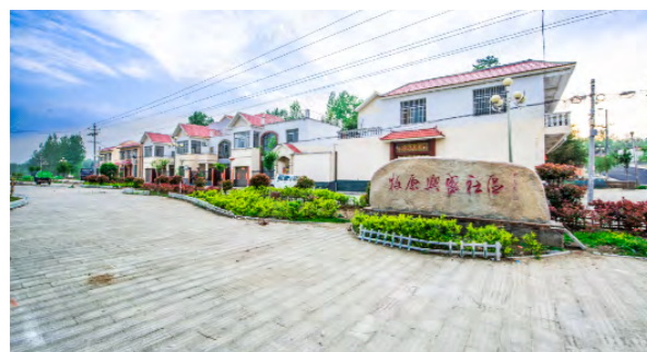
Community infrastructure constructed with help of Neixiang MUYUAN (Henan Province)
