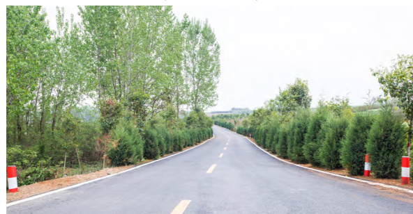
Assistance in road construction for local community by Neixiang MUYUAN (Henan Province)
