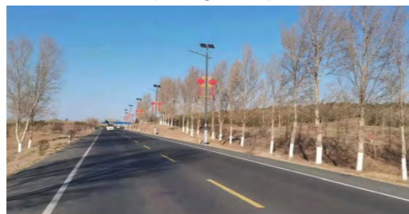
Street lights installed with help of Aohan MUYUAN in Inner Mongolia
