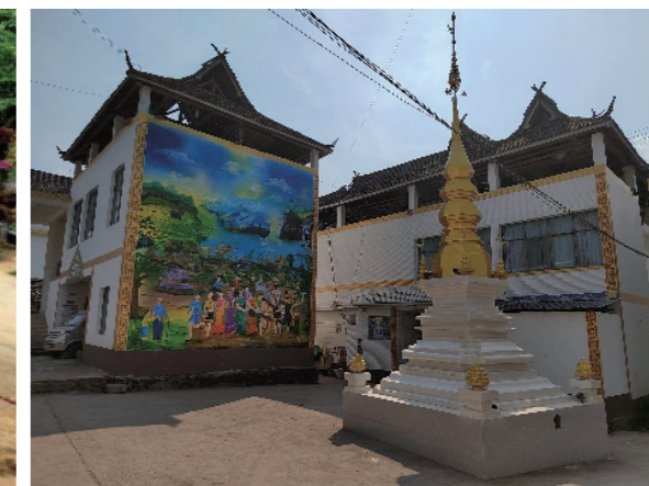
Photo of a rural leisure resort project in Likan, Mengsuo town, Ximeng County
