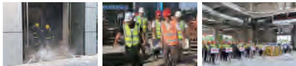
CDF Investment Development carried out firefighting emergency drills CDF Investment Development carried out struck-by emergency drills for projects under construction CDF Investment Development carried out firefighting emergency drills for projects under construction
