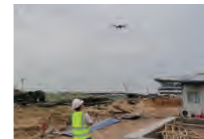
Using drones to inspect the construction site
