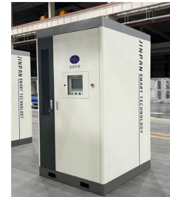
233kWh modular commercial and industrial energy storage unit
