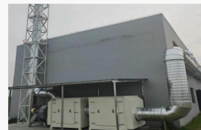
This year, Carpoly's Anhui plant upgraded its hazardous waste and water treatment areas to collect unorganized exhaust gases, reducing non-methane hydrocarbon emissions. In 2024, the water treatment system operated for 2,392 hours, reducing emissions by 227 kg of non-methane hydrocarbons, 62 kg of ammonia, and 4 kg of hydrogen sulfide.
