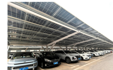
Installation of PV Canopies in Employee Parking Lots
