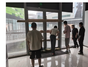
▲ Reinforcement of doors and windows at the Riyue Plaza Duty-Free Shop
