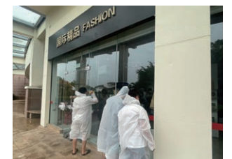
▲ Reinforcement of doors and windows at the Boao Duty-Free Store
