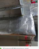
Fireproof Wrapping and Soundproofing Setup for the Static Pads for Fan Units
