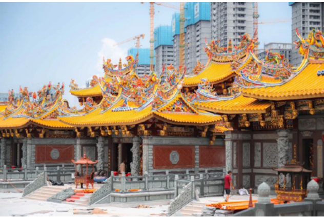
钟宅古民居修缮
