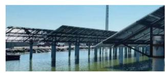
High-corrosion-resistant weathering steel for marine photovoltaics supplied to Huaneng Binzhou 850 MW photovoltaic power project.
