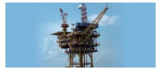
High-strength steels such as DH36 and EH36 applied to jacket structure of the Liuhua 11-1 platform.
