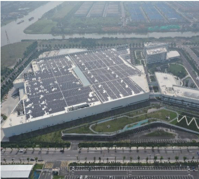
南通富创屋顶光伏
