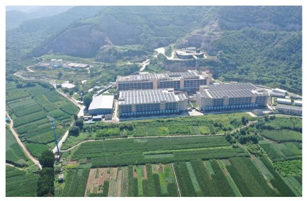
Photovoltaic installation on multi-story pig farms
