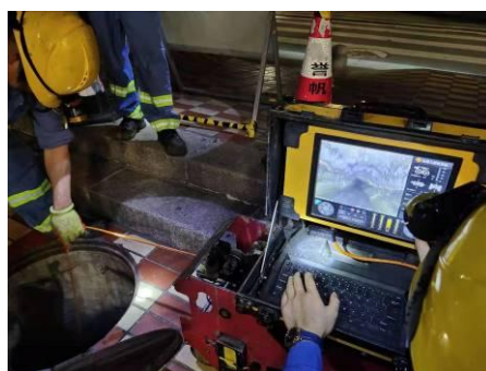
宜宾翠屏区检测现场
