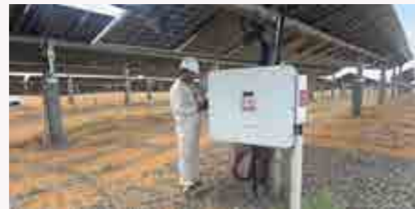
■ On-site Commissioning and Maintenance
