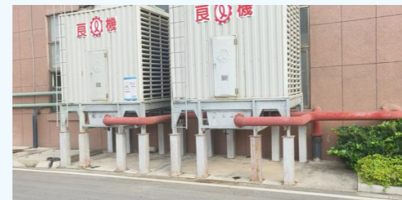
Facilities for recycling equipment cooling water
