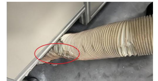
Deformed pipe in an environmental facility
