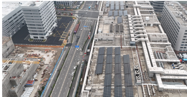
Construction of the 399.26 kW PV project at the Ningbo Beilun 246 Base
