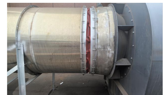
After pipe repair
