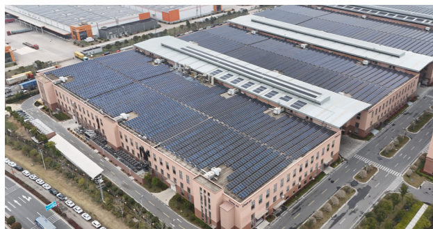
Construction of the 6 MW PV project at the Ningbo Longshan Base
