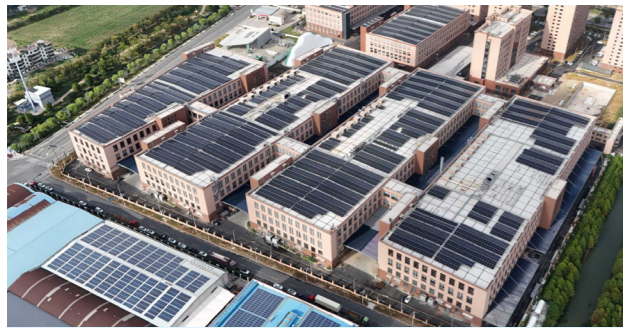
Construction of the 5.88 MW PV project at the Haiyan Base
