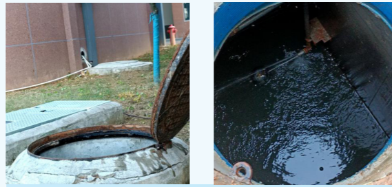
Rainwater storage reservoir
